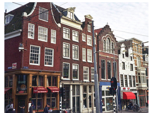
The houses at the corner of Vijzelgracht and Prinsengracht were among the early tracts restored by the Stadsherstel
