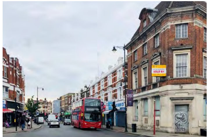
Harlesden High Street, London. A former bank building renovated as an education center by the Refugee Support Network
