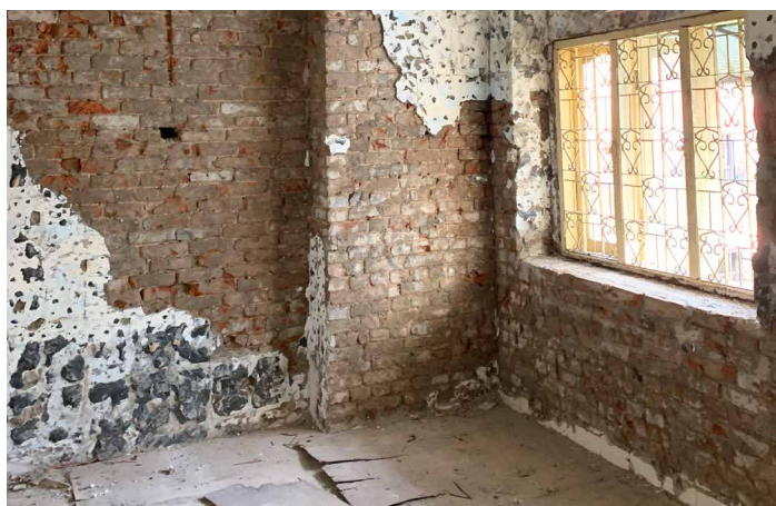
Example of heritage house interior before and after restoration
