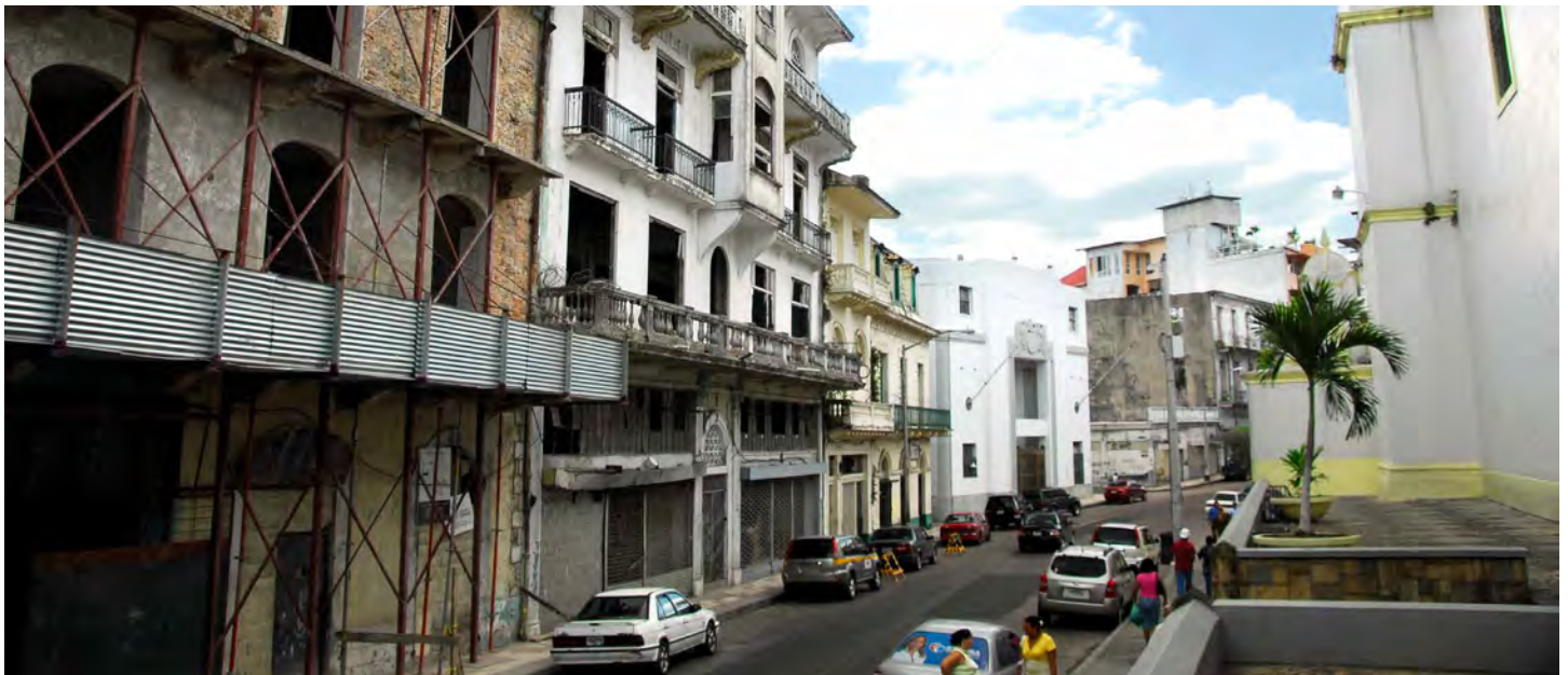
Panama City, ongoing building restorations in Casco Viejo
