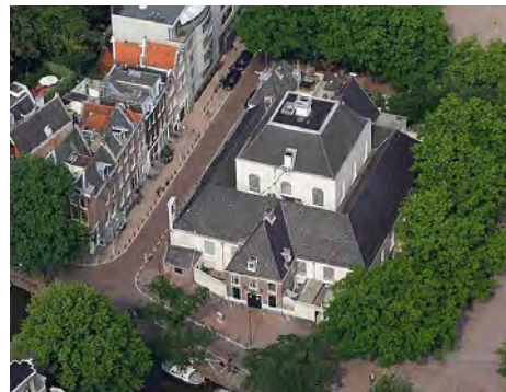
In recent years the Stadshertel has taken on the conservation and adaptive reuse of landmark buildings, such as the Amstelkerk, now the headquarters of Stadsherstel.
