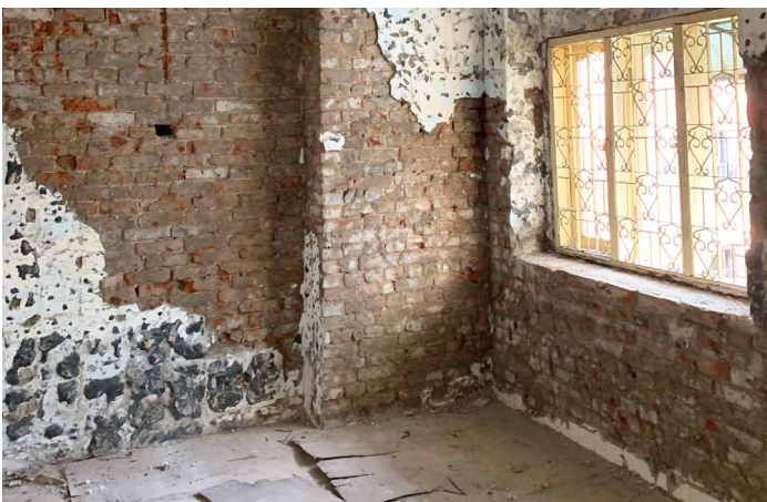
Example of heritage house interior before and after restoration
