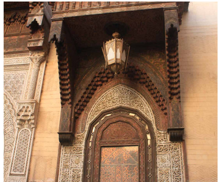
Examples of plaster and wood work embellishment of houses and other structures restored using traditional techniques.
