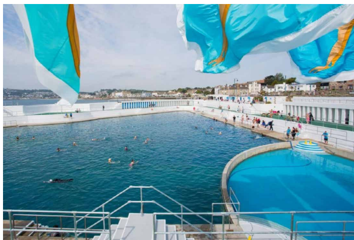
Jubilee Pool, Penzance (Cornwall), England, general view
