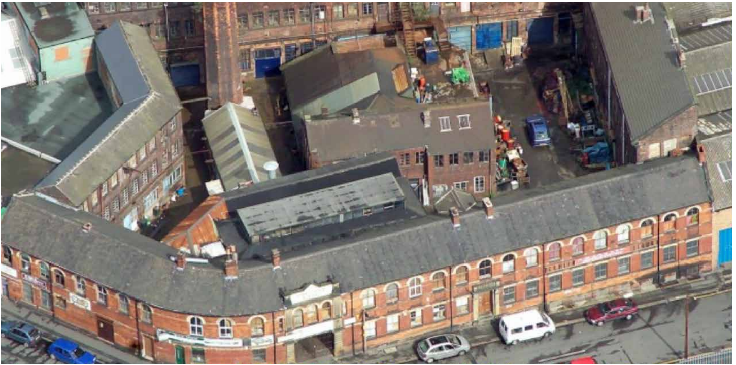
Portland Works, Sheffield (England), aerial view
